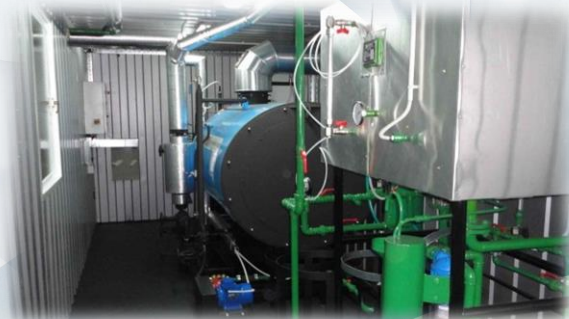
AFROTROPIC COCOA PROCESING Co. Ltd., Gana Steam container boiler room, 600 kg /hr - 12,6 bar
