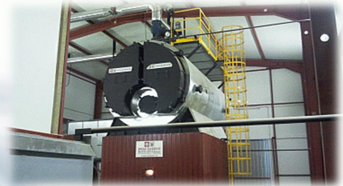
MMM VUKELIĆ Hot water boiler 4MW, sawdust
